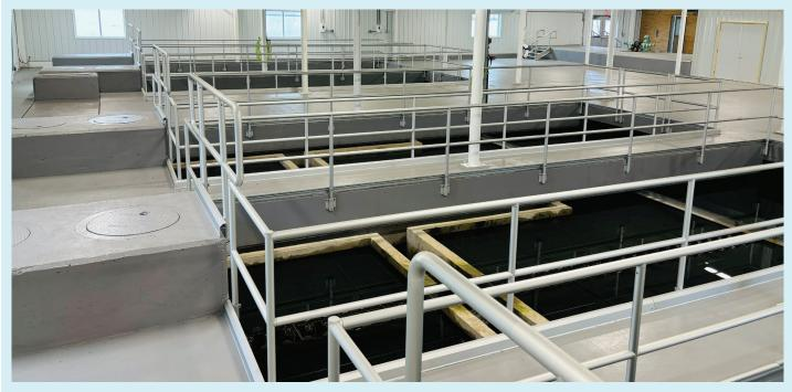
The Huron Water Filtration Plant produced over 888,000,000 gallons of drinking water in 2023. This equates to an average of 2.4 million gallons of drinking water per day provided to the City of Huron and surrounding Erie County. The filtration plant draws water from Lake Erie and it is then purified by a conventional treatment process. This process consists of coagulation, flocculation, sedimentation, filtration, and disinfection. (Pictured: Sedimentation Basins)
